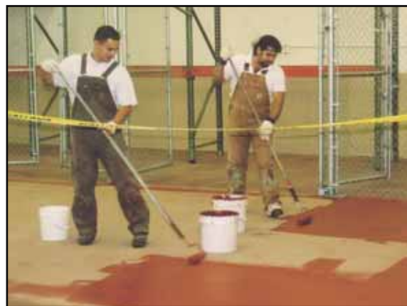
Left: Broadcasting aggregate onto EPI's coatings provides a textured, non-skid finish for wet floors.
