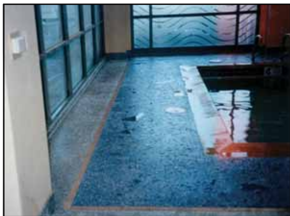
Left: Broadcasting aggregate onto EPI's coatings provides a textured, non-skid finish for wet floors.
