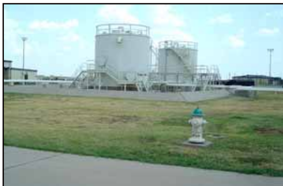
This military base selected an EPI Coatings System to create a safety barrier between hazardous materials and the environment.
