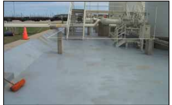
Grit is applied to EPI Quick Set Epoxy to provide a textured, skid-resistant surface.
