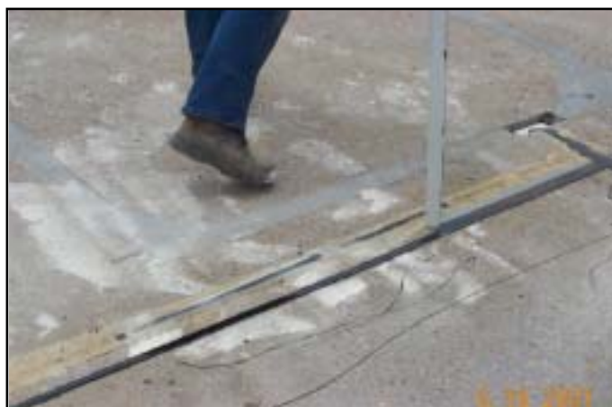
Joint Seal works over a wide temperature range, sealing in minutes, with no damage to traffic sensors
