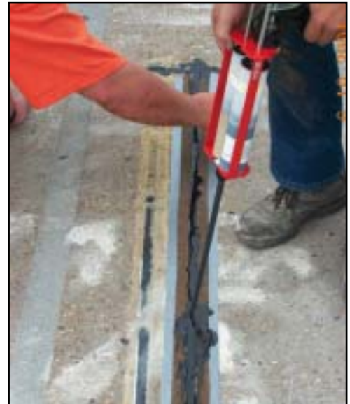
Highway employees use Reactamine® Joint Seal to install piezoelectric axle sensors
