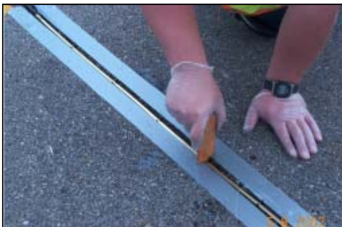
Highway employee lays out a sensor to count, classify and weigh vehicles.
