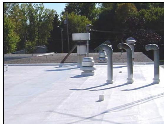
EPI created a single coat, superior aromatic, SMP coating for roofs. It replaces a dual coat system.
