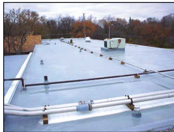
SMP roof coatings provide superior waterproofing through a full-adhered, seamless and elastomeric barrier. Photos: Crown Fluid Applied Systems
