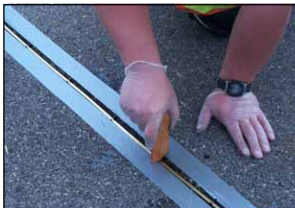
Highway employees use EPI Joint Sealant to install piezoelectric axle sensors
