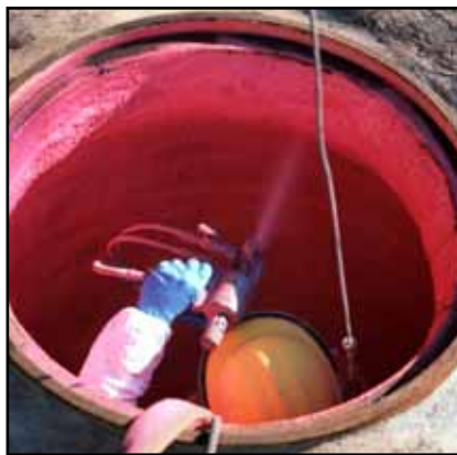
EPI's silicone-modified coatings stop manhole water infiltration, structural deterioration, and corrosion problems
